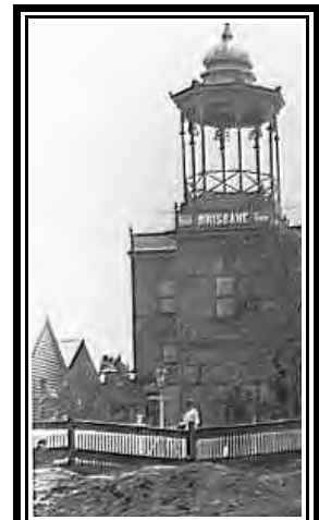
Another view of the German Club showing part of the east end of the Roemermann house. Part of a photo from the State Library of Queensland.
