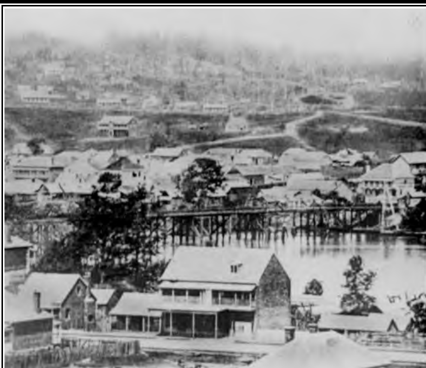
The first Victoria Bridge - opened 1865 - Looking from the city towards South Brisbane. John Oxley Library Image No. 147690.
