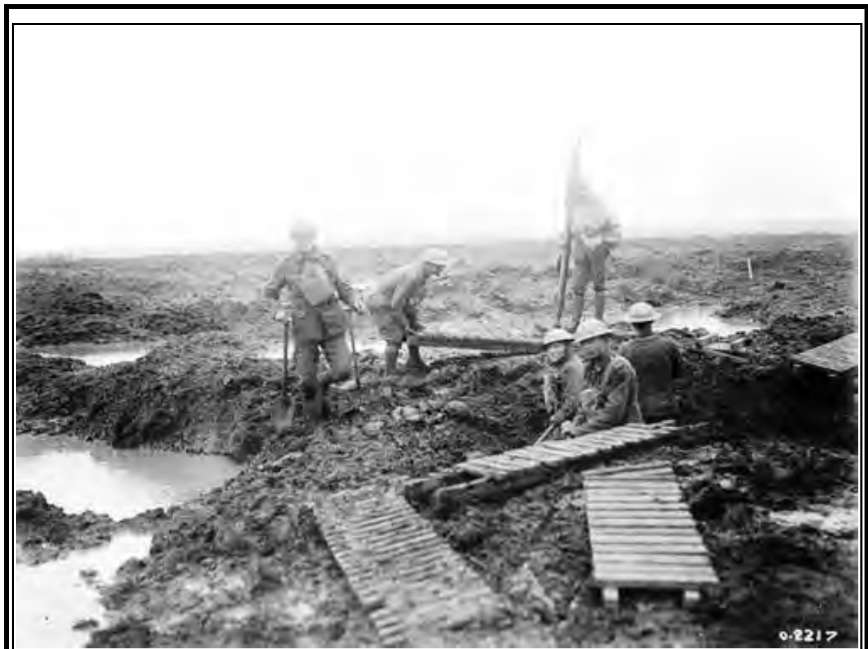
Canadian Pioneers laying trench mats over mud, Battle of Passchendaele. Photo from William Rider-Rider/Canada. Dept. of National Defence/ Library and Archives Canada/PA-002156.
