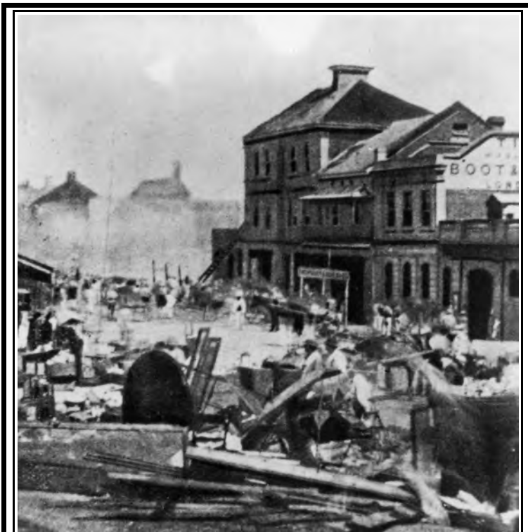
This view was taken looking south towards the river from near the Albert Street corner. Compare with the previous photo on page 75 taken before the fire. Photo courtesy of Brisbane City Archives.
