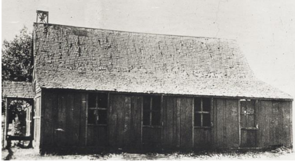
St Luke's original slab hut schoolroom, built 1857 [John Oxley Library, State Library of Queensland, neg. 36932]
