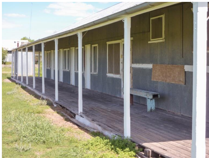
Shearers' quarters, Wyaga Station, constructed of timber slabs [John Field, 2014]
