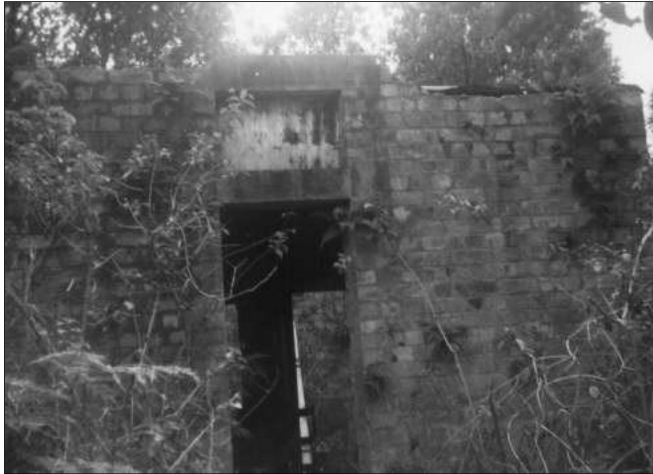
"Cell Block", The Bluff, Peel Island, 1990s
